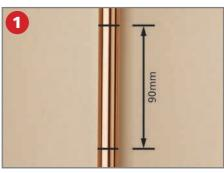
Drain the central heating system or plug-off feed and expansion tank and release the system pressure. Measure and mark a 90mm section when making the connections with elbows supplied, as shown in step 3 below. When installing below a boiler or other object, allow 170mm clearance from the top of the canister to beneath the object, to enable the lid assembly to be removed when servicing.
