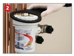
Using the MagnaClean Micro lid spanner, carefully unscrew the lid.
