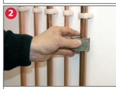
Using a suitable cutter, carefully remove the marked section of pipework to create the correct opening.
