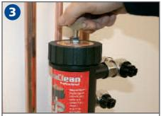
Replace the Pro-Fill air vent. Allow the system to circulate for 30 seconds. Open the Pro-Fill screw two turns and back flush until clear.
