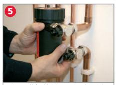
Loosen off the valve flange nuts and insert the rubber washers provided. Thoroughly tighten the flange nuts. Do not over tighten.
