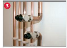
Prepare the pipe and fittings accordingly. Lubricate the olives and assemble the valves on the pipe. Hand tighten.
