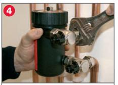
Loosely secure the MagnaClean Professional canister to the valves. Grip the MagnaClean canister and tighten the compression fittings being careful not to over tighten.
