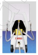
2c. Across the "tails" of a radiator (having drained and disconnected the radiator) using appropriate 1/2" or 3/4" BSP adaptors to connect to the valves. The radiator valves should be closed to isolate the flushing pump from the system until power flushing is commenced.
