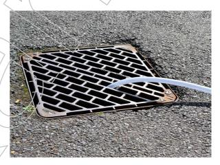
5c.The mains water inlet supply (orange tap) should now be turned on and adjusted so that the volume of incoming water compensates for that being forced out of the system to waste. Continue dumping until the waste water runs relatively clear. Ensure that the water level in the tank remains at least 10 cm above the minimum mark at all times.
